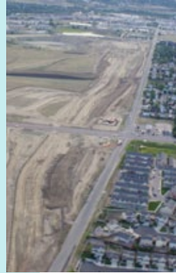
August 2010 aerial photograph Milton E. Proby Parkway construction
