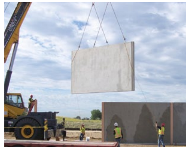
Unloading and placing concrete sound walls.
