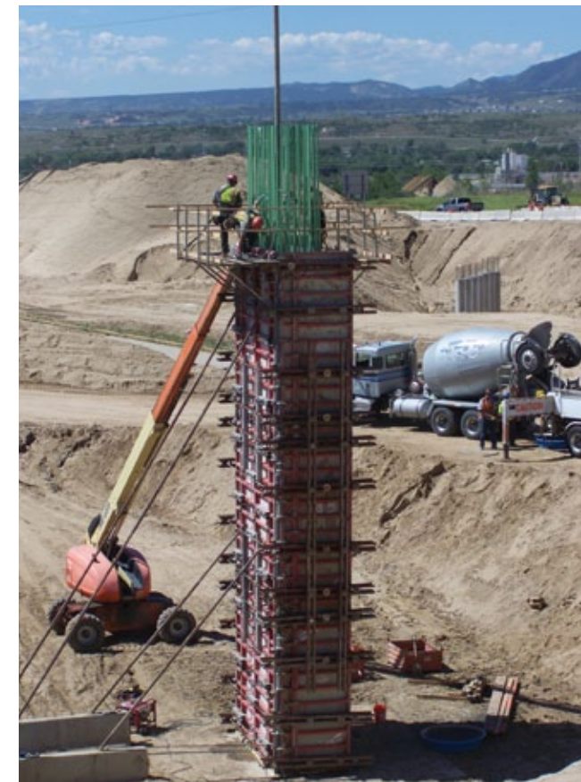
Pouring Concrete for Pier 6 on Ramp C.
