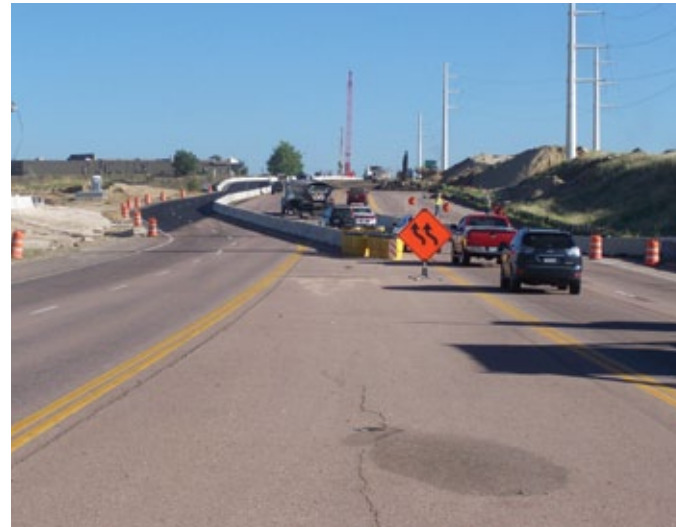
Academy Blvd. lane shift.
