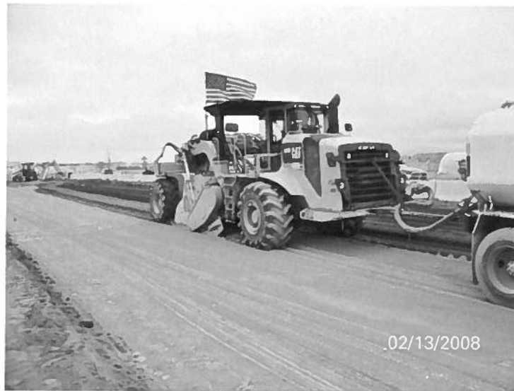
Subgrade Stabilization
