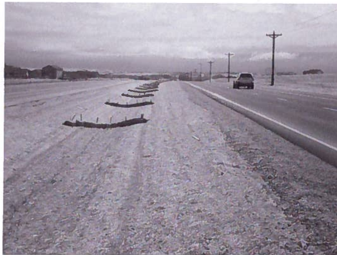
New Southbound lanes looking South
