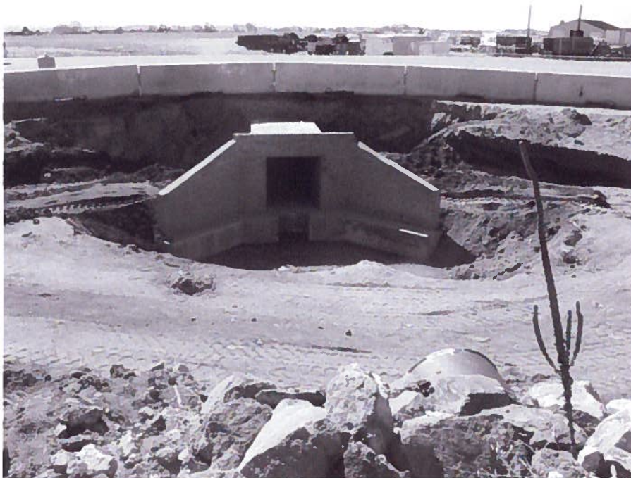
HWY 24 Box Culvert Extension
